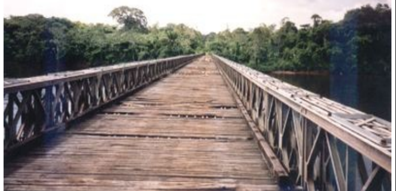
A “single triple” bailey bridge
